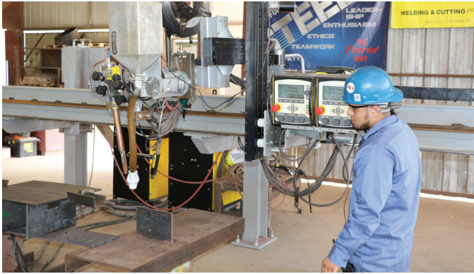
Fig. 3 — The side-beam mounted SAW system can weld joints up to 25 ft long, increasing Patriot Erectors' competitiveness when bidding on structural steel projects.
