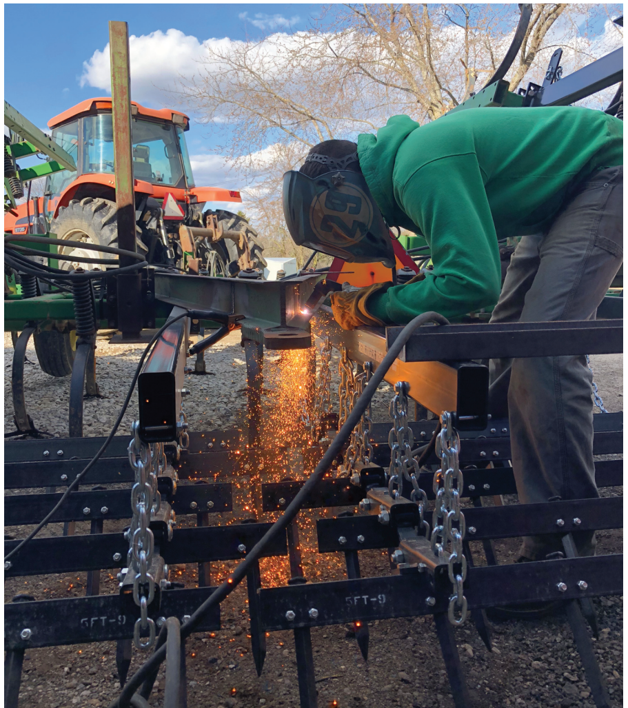
Fig. 1 — Justin Sly modifies farm equipment. He is pictured here removing hangers on a rolling basket so rakes can be added to this soil-cultivating machine.
