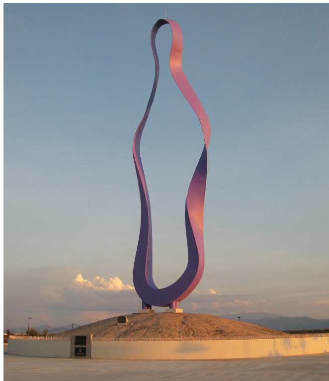
Fig. 6 — El Manto de la Virgen (Virgin Mary's Veil). A 100-ft.-tall religious monument commissioned for the city of Torreon, Mexico, made of carbon steel using GMAW and SMAW, and finished with enamel paint.
