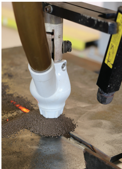
Fig. 5 — In a single-wire configuration on a 0.625-in. steel tube, the SAW system can deposit up to 20 lb of weld metal per hour with a 5/32-in.-diameter metal-cored electrode.
