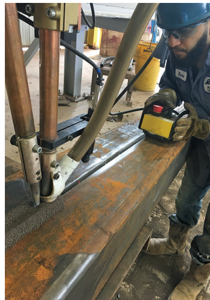
Fig. 6 — Switching to a narrow groove angle for the canopies reduced filler metal use by 17% and boosted SAW productivity.
